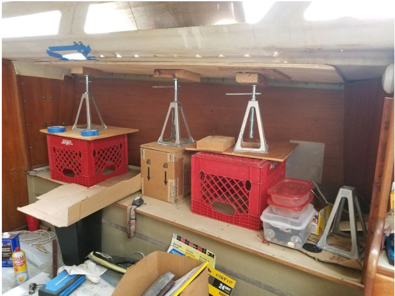
Adjustable screw jacks used to support the starboard side deck while working on it. Installed before cutting the top skin out of the deck, this trick supported all the weight used to bond the top skin back on and key to getting the final shape to match.
