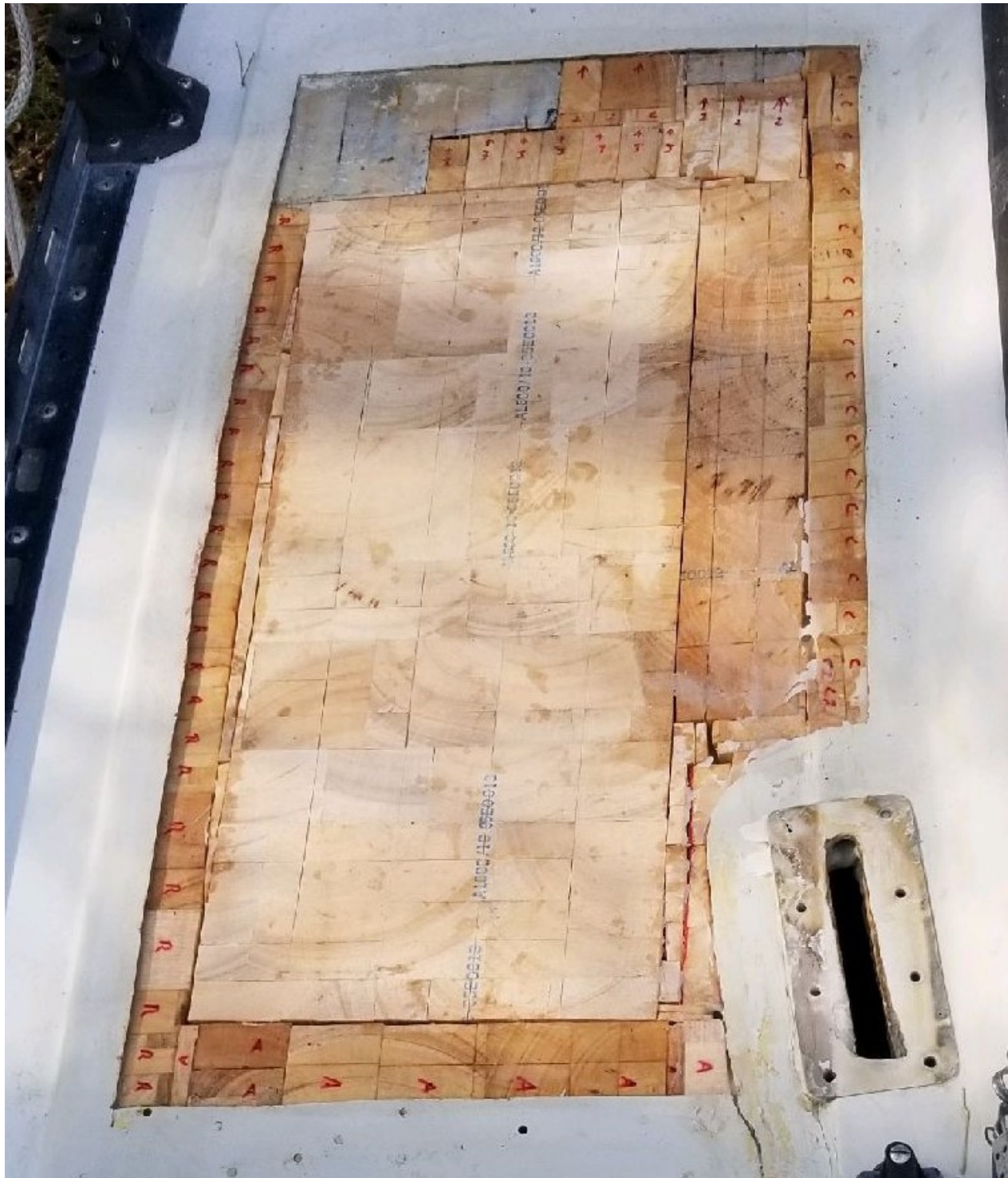
Port side; new balsa dry fitted. Some pieces were marked for location because they got brushed with epoxy and stuffed into the void around the perimeter. These were all epoxied in place before fitting the larger center rectangle of balsa. All voids were filled with West System epoxy thickened with 404
