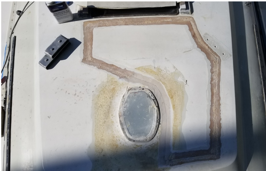
4) 12:1 bevel ground along joint
