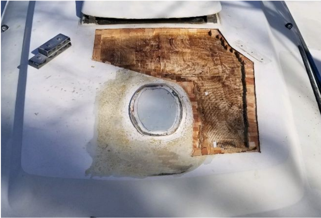
1) Old core removed, new core going in.
