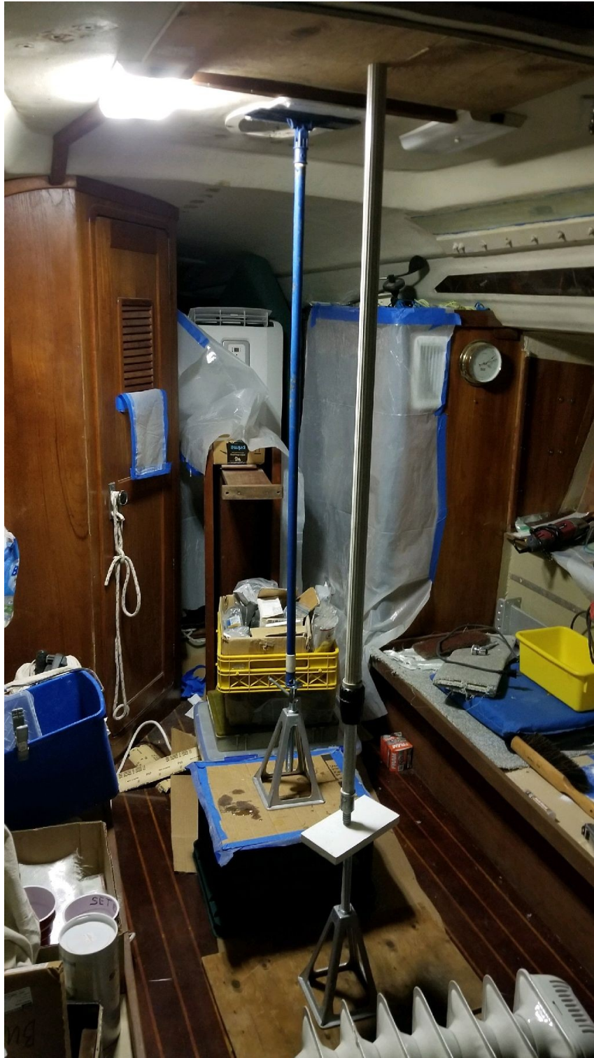
Supporting the cabin top and maintain a proper camber while repairs were made above. Adjustable painter's pole, a swifter mop and a screw jack.
