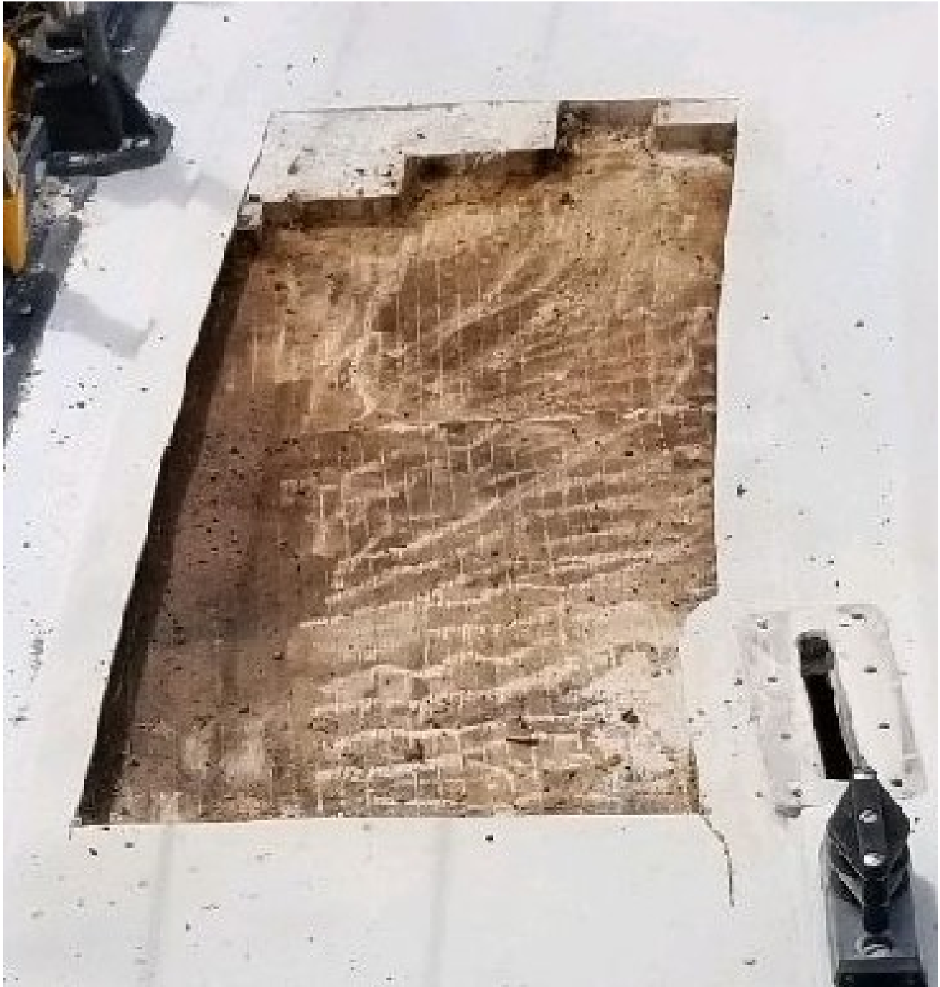
Port side balsa removed
