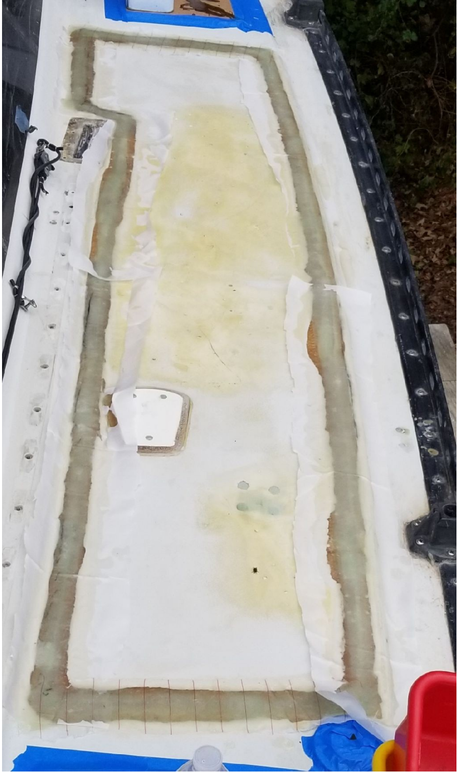
Starboard side; two layers of 1708 epoxied into bevel, covered with peelply
