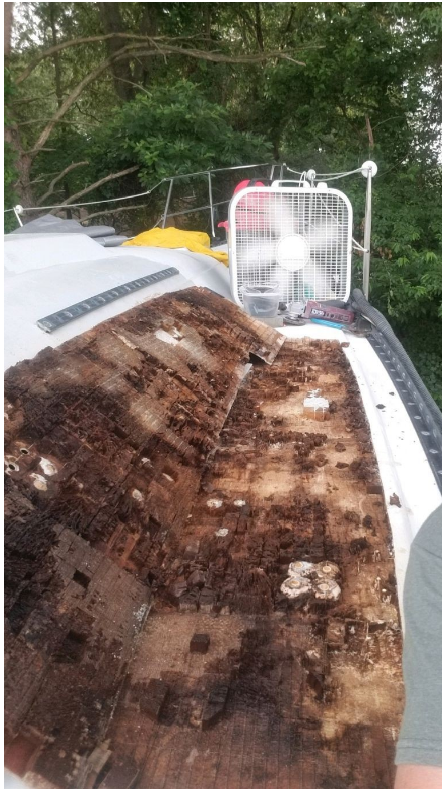
Starboard side; top skin removed showing wet balsa
