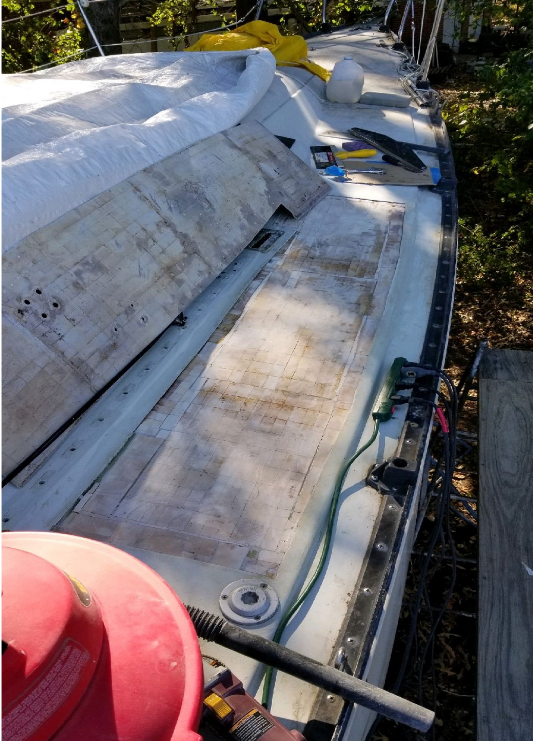
Starboard side: New balsa installed, sanded and ready for top skin
