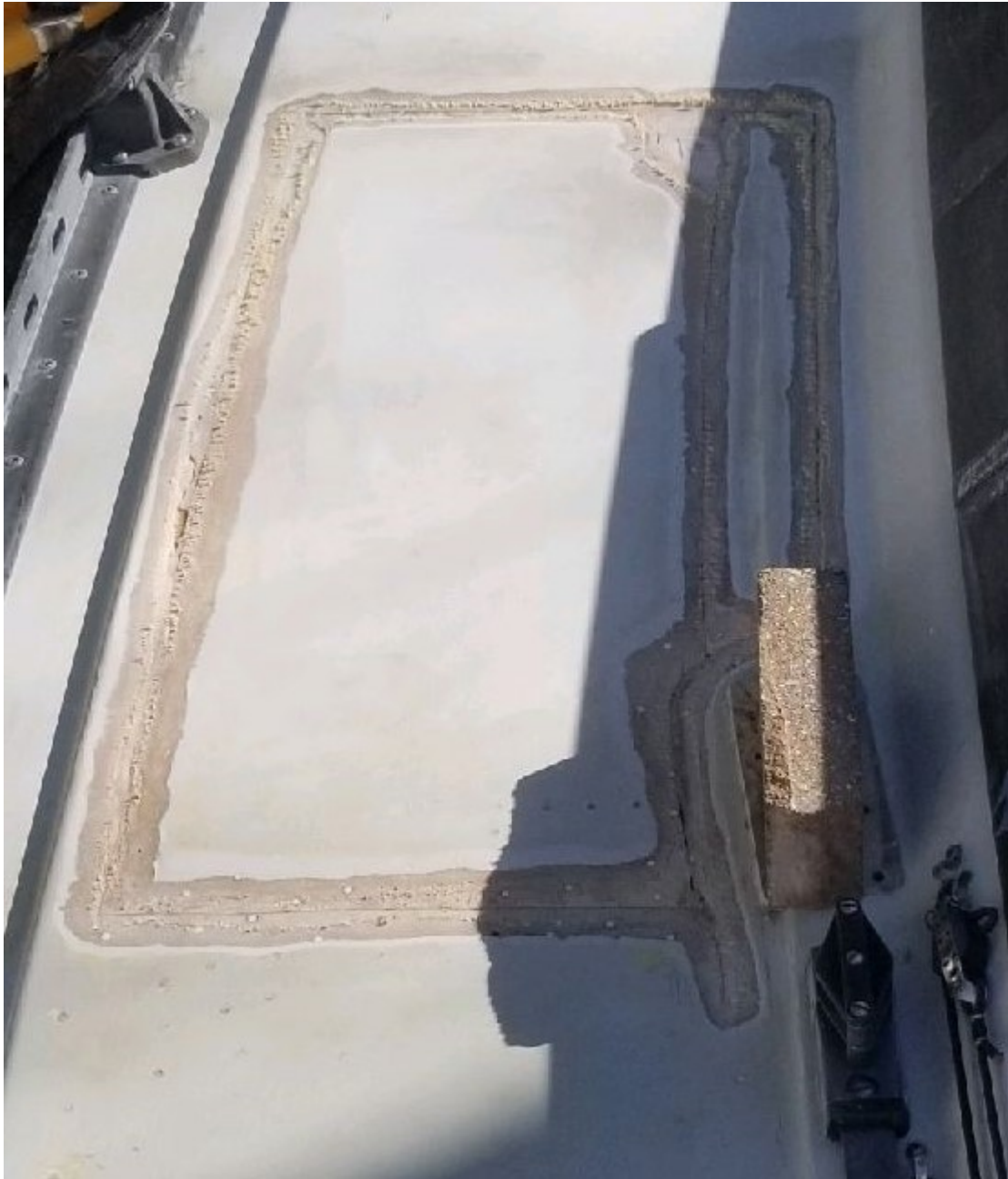
Port side; joint ground down to 12:1 bevel
