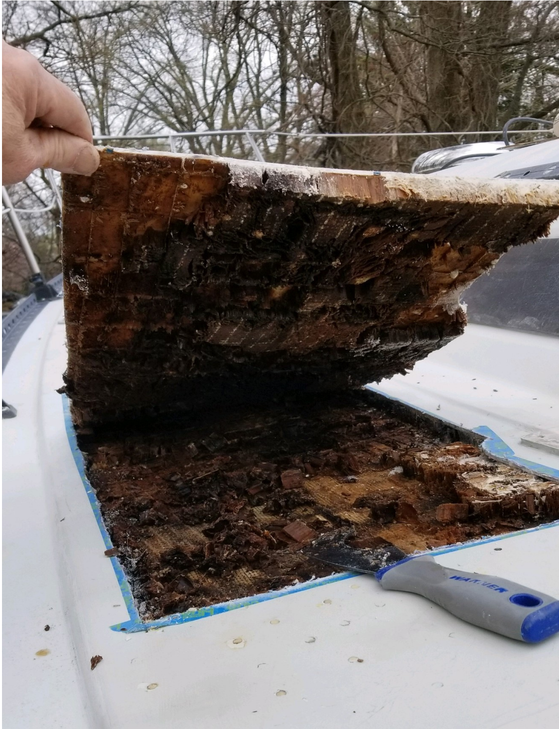
Port side deck; skin lifted showing wet balsa core
